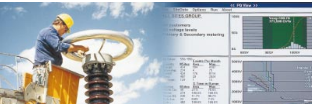
Voltage divider being erected for staged fault testing in a substation. Data is used to evaluate circuit breaker performance.
