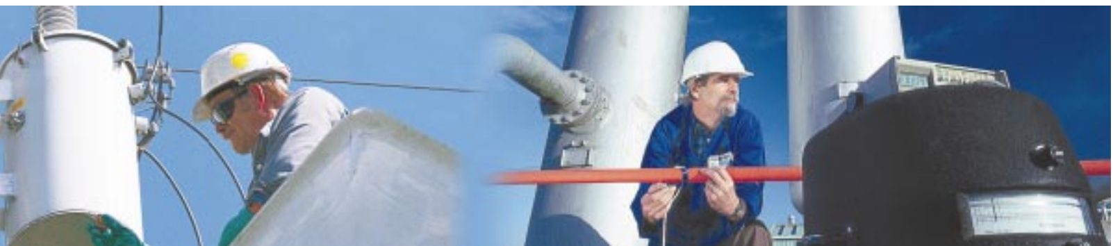
Sample of transformer oil being removed by client for delivery to Powertech to test for PCB content.
